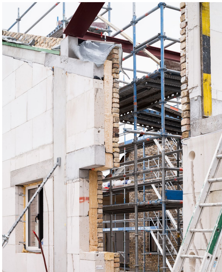
2025 – photograph made on a construction site in Lokeren, BE.
